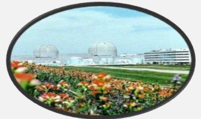
South Texas Project
