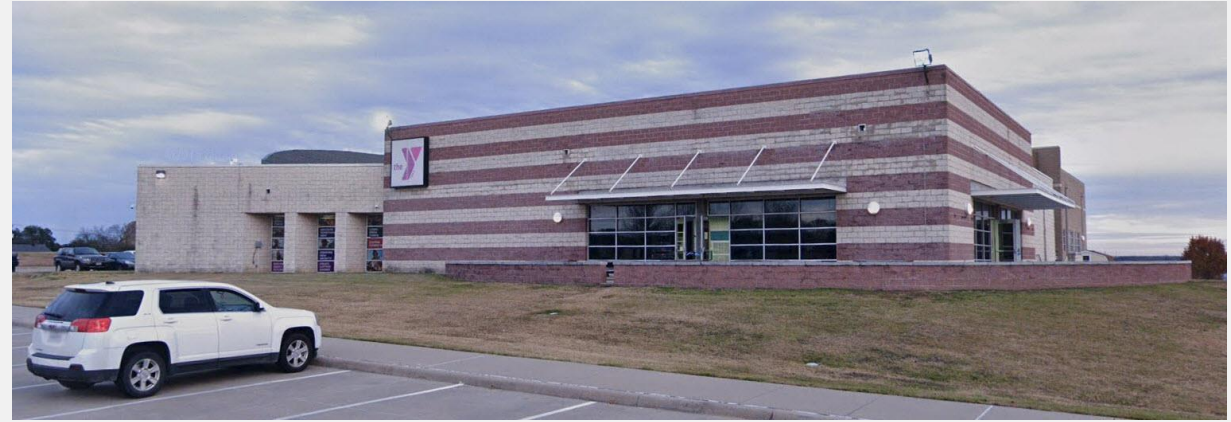
Assembly Area for CRC Processing
