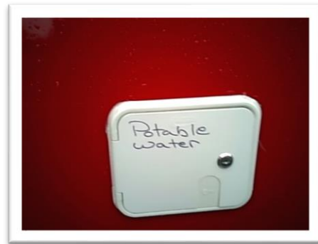
Potable Water Inlet
